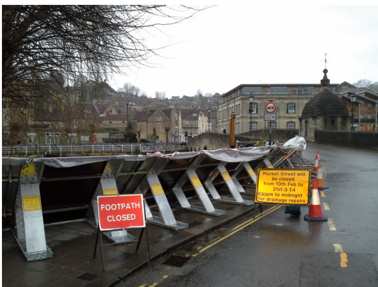
In 2014 Wiltshire Council worked with the Environment Agency to install temporary flood barriers to help protect Bradford on Avon from flooding from the Bristol Avon.
