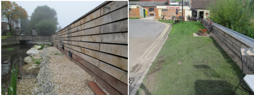
At Marlborough a flood alleviation scheme was jointly funded by the Environment Agency, Wiltshire Council and Marlborough Town Council.
